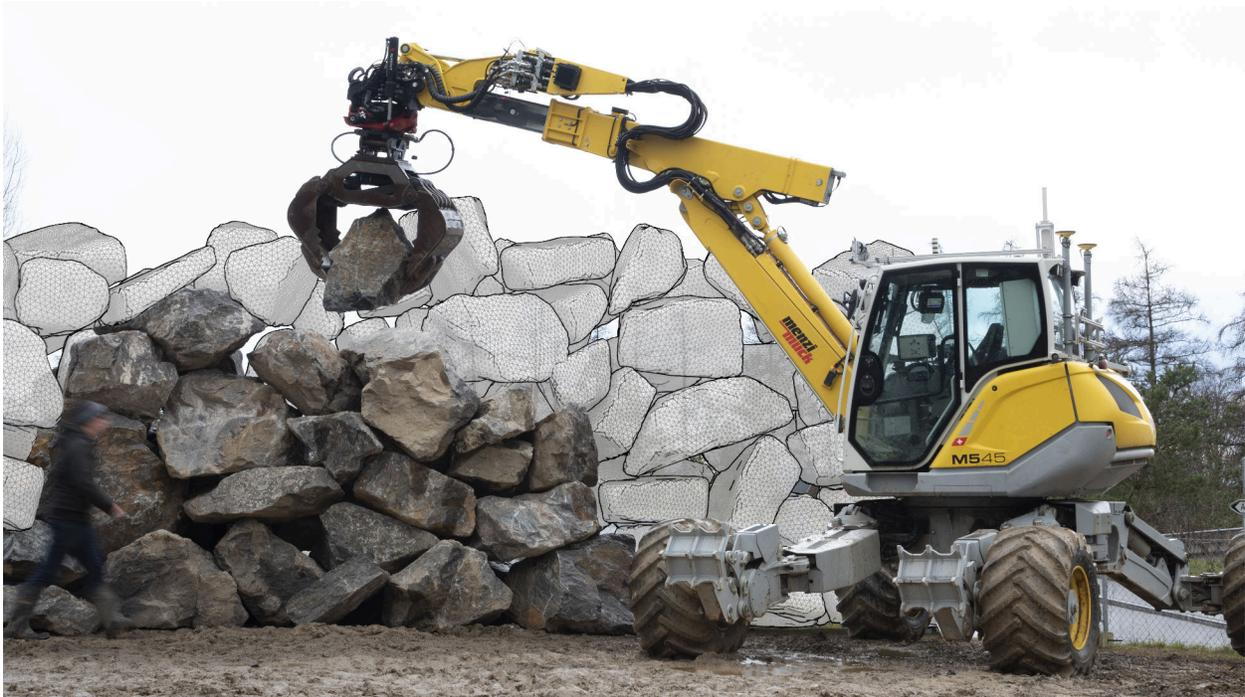
Figure 12: The presented mapping and manipulation tools in this paper were used for the application of dry stone wall construction with the autonomous hydraulic excavator HEAP. The in-progress wall is overlaid with a potential extension of the structure, generated by allowing the geometric planning to continue with additional digital stone models. Further details on the geometric planning of the desired stone poses can be found in (Johns et al., 2020).
