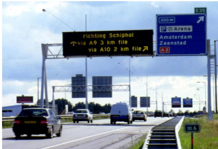
Figure 9: A route guidance system in The Netherlands showing traffic jams lengths on alternative routes to Schiphol Airport. (Photo courtesy of Peek Traffic B.V.)
