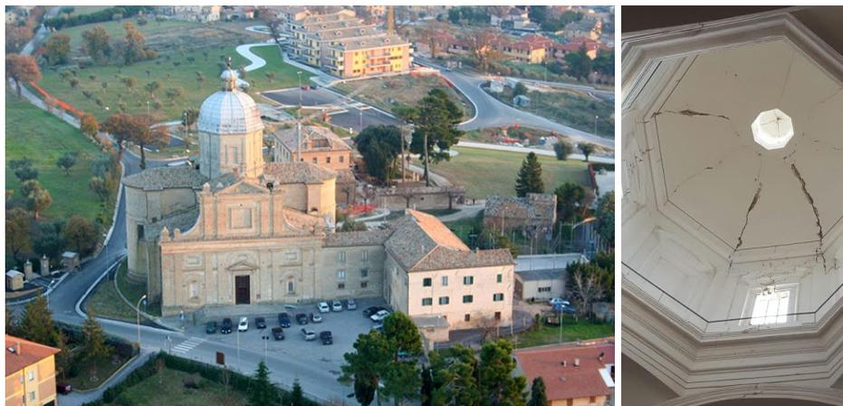
**Fig. 1.** - Aerial photo of the church of Santa Maria delle Vergini in Macerata before the 2016 earthquake (on the left) and the dome damaged in 2016 (on the right).
