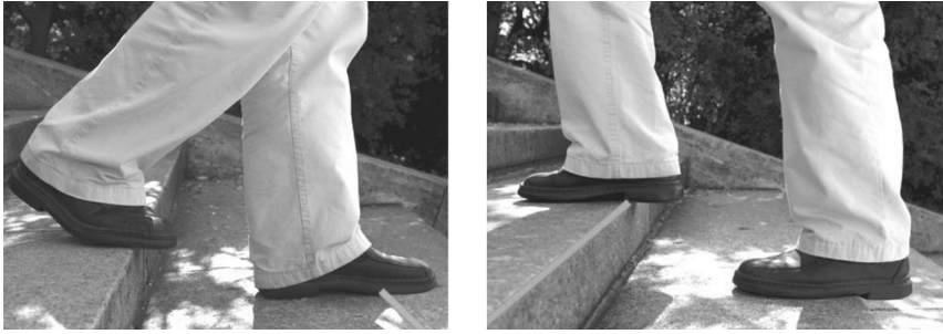
Fig. 3. Sensory role of the foot while walking up and down the stairs - overhanging heel or nose of the foot over the below tread of stairs enables to locate position edge of the step. (Photo: M. Pelczarski).
