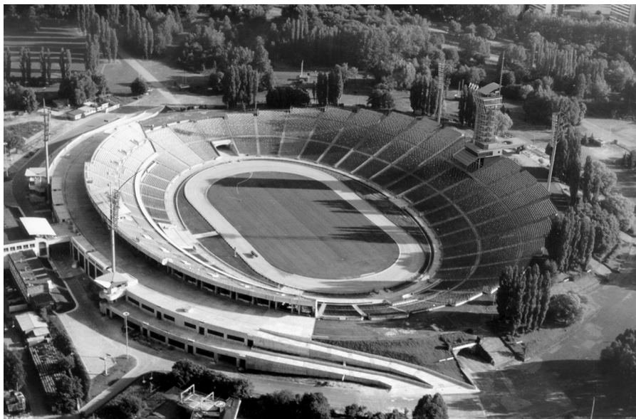
Fig. 10. Located in a 600 ha urban park, Silesian Stadium in Chorzow, Upper Silesia, Poland (the state after redevelopment 1994–2007). Two pairs of wide ramps, North and South, in time shorter than 5 min, are able to evacuate all viewers from this part of stadium directly to the main exit gates. (Source: Archives of WOSiR, photo - P. Oles).
