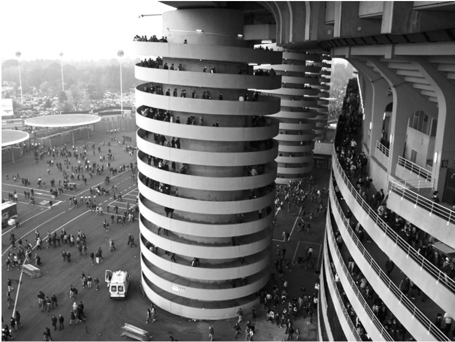
Fig. 11. Efficient and spectacular spiral and peripheral ramps serving the circulation and evacuation movement at the San Siro stadium in Milan. (Photo: Timothee Nalet, http://www.timotheenalet.com/urban/milan-san-siro , admit. 2015-02-15).
