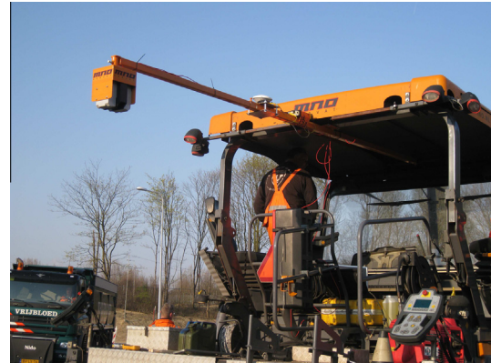
Fig. 6. Linescanner mounted behind a paver.
