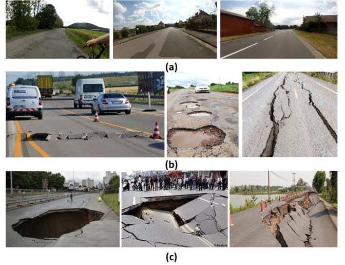
Figure 6: Image examples of abnormal roads in (a) Low level, (b) Middle level, (c) High level.
