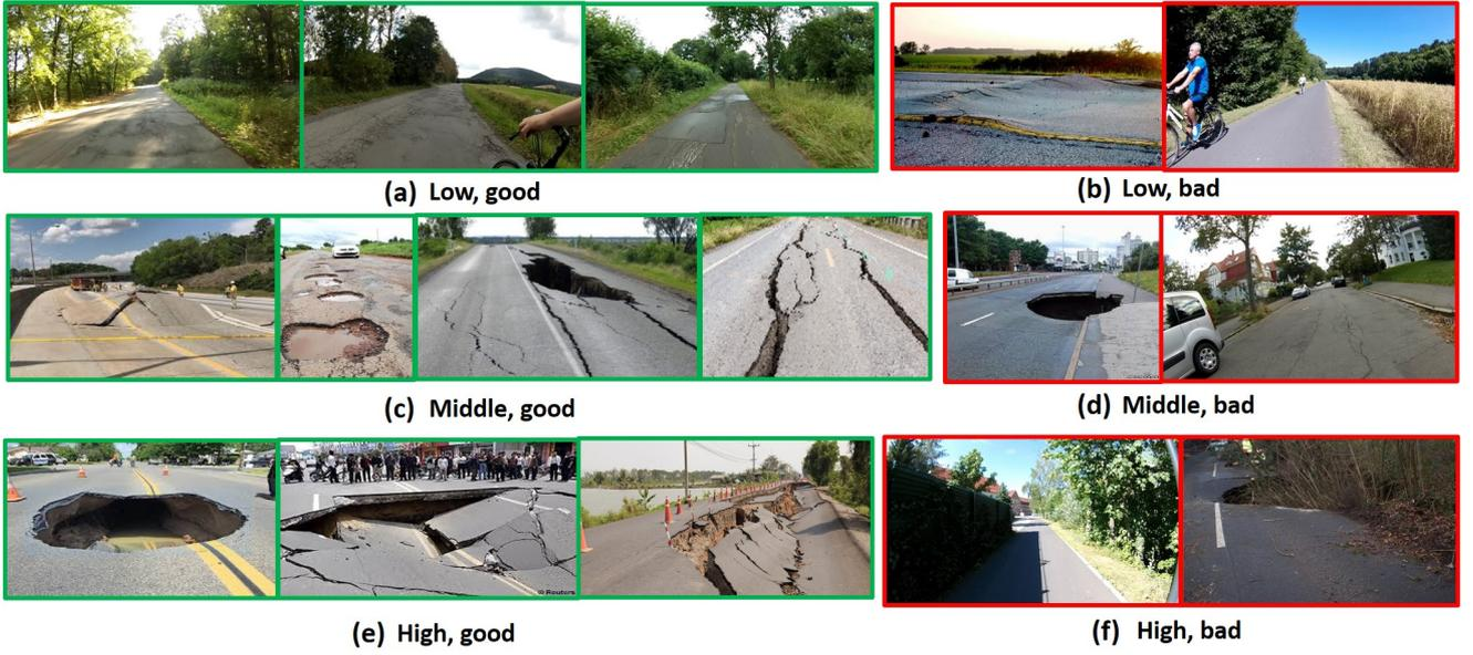
**Figure 8:** Experimental results of the ADD model. (a) Good results of low-level road damages, (b) Bad results of low-level road damages, (c) Good results of middle-level road damages, (d) Bad results of middle-level road damages, (e) Good results of high-level road damages, (f) Bad results of high-level road damages.
