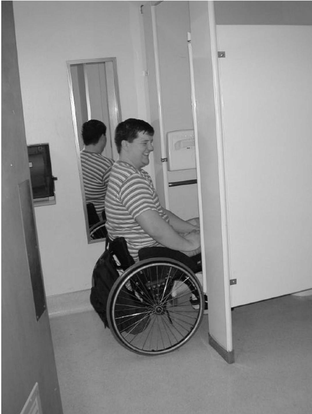
Fig. 23. Inaccessible water closet. The photo shows that a wheelchair user is unable to access the men's toilet in the facility diagrammed in Fig. 21 and referenced in Fig. 22.
