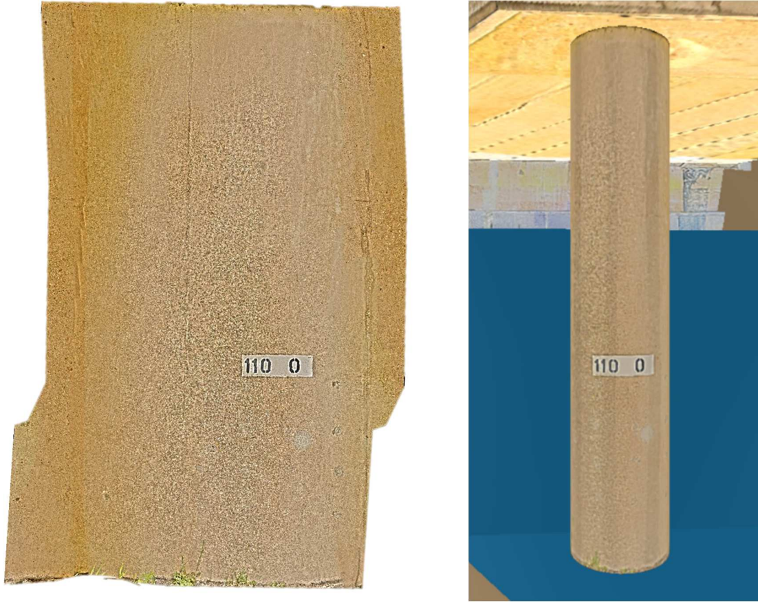
Figure 4: Reconstructed high-resolution surface texture of a bridge column, uncoiled 2D view on the left, 3D view on the right
