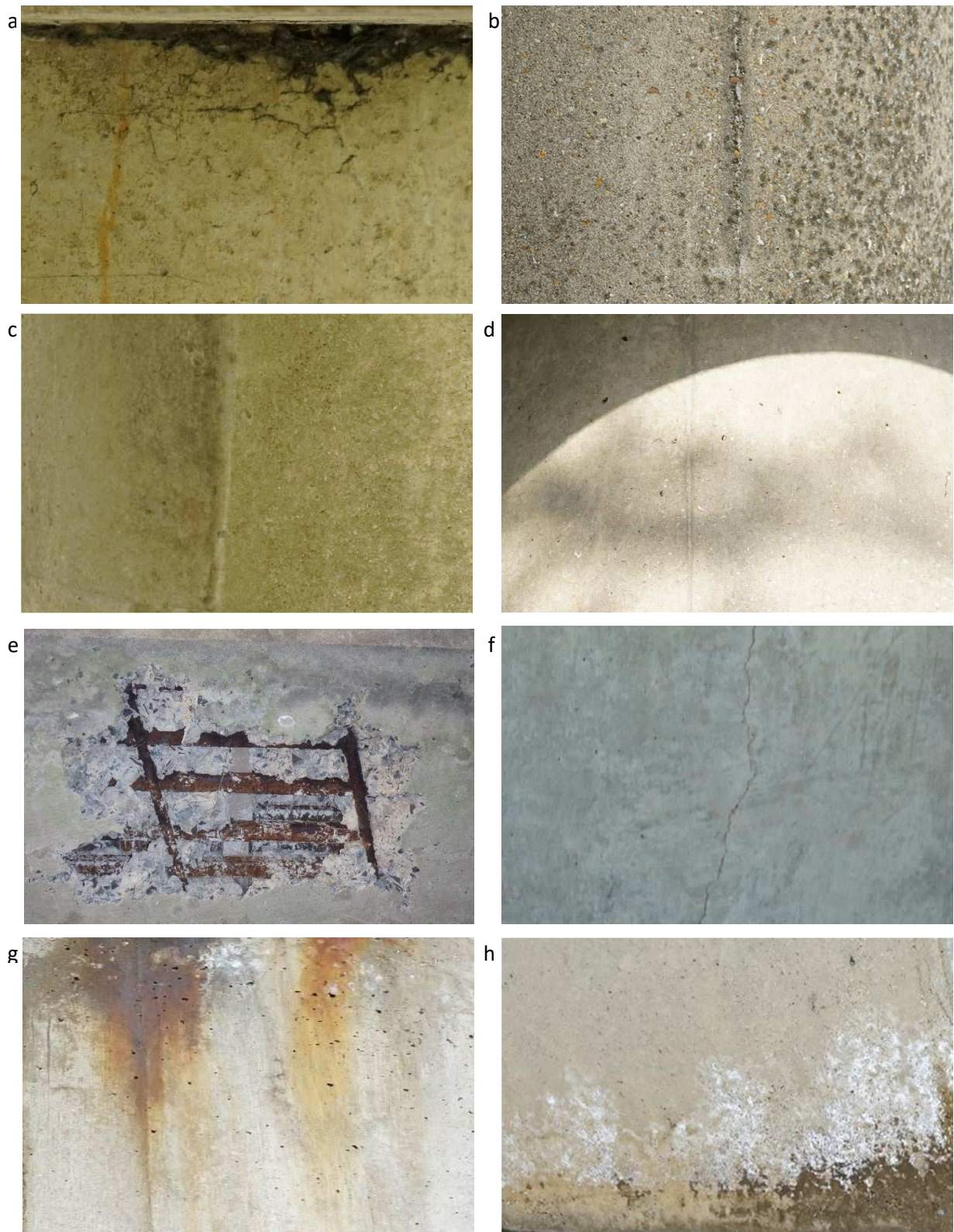
Figure 2: Concrete texture examples: (a) dust, dirt and spider webs, (b) formwork marks, (c) water stains, (d) strong shadows, (e) spall, (f) crack, (g) rust stain, (h) efflorescence
