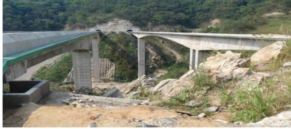
Figure 5: Three-span Continuous Rigid Frame bridge (TCRF Bridge).
