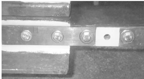
Figure 2: Arrangement of rail feeding terminals
