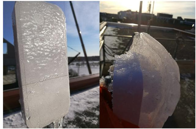
Fig. 12. Link front part covered with ice in winter time.
