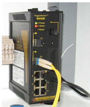
Figure 7 Ethernet Switch Installed in the Substation Control Room
