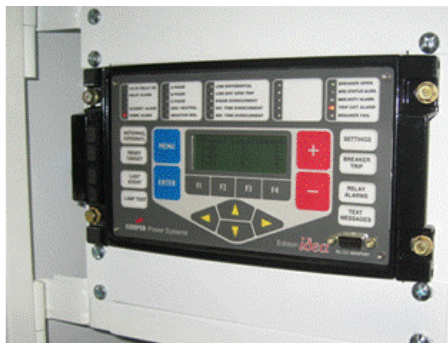
Figure 6 Relay Installed in the Substation Control Room
