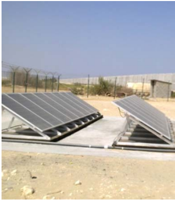
Figure 5. 5kW PV array at KFUPM beach, Dhahra, Saudi Arabia
