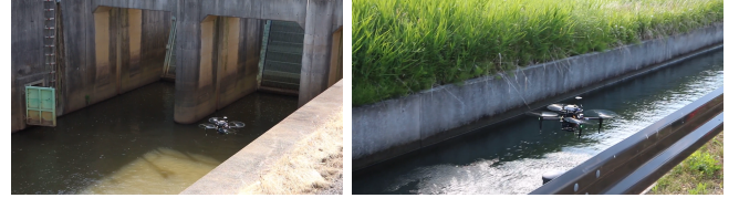
Fig. 1: UAV taking photos of water canals for damage assessment
