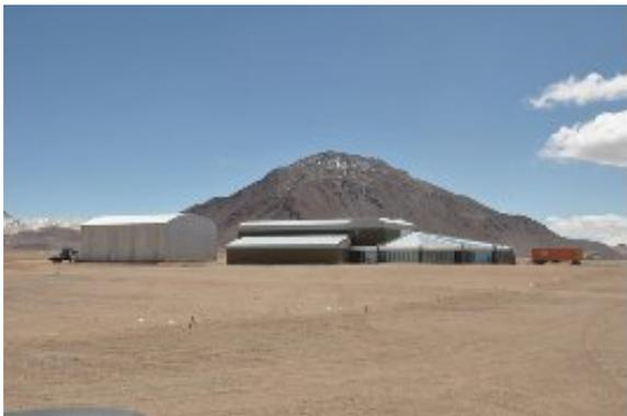
Fig. 7. The Array Operations Site Technical Building houses the correlator and the Local Oscillator System. At 5000 m elevation, it remains unstaffed most of the time.
