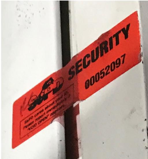
Fig. 7: This style of seal is used throughout a municipality. In order to identify whether the correct seal is being used, consumers must be aware of the type of seal expected to be present.
