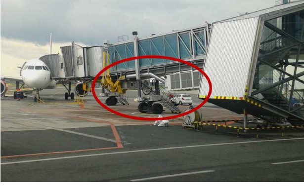
Fig. 7. A jet bridge containing an embedded air conditioning system.
