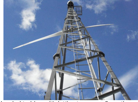
Fig. 4. Gaia wind turbine with lattice tower configuration
