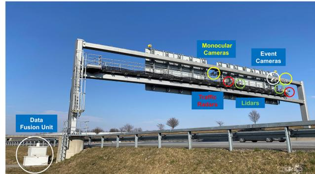
Fig. 1. One of the measurement points on the highway A9 from Providentia++ project (<https://innovation-mobility.com/en/project-providentia/>).
