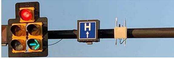
Fig. 12: The roadside unit at the intersection. Photographed by City of Dublin [47].
