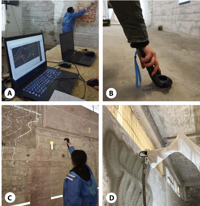
Figure 5: (A) Selection of filter (B) localization (C) designing, adjusting the design (D) robotic spraying.
