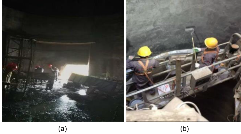
Fig. 3. Working conditions at the bottom platform of the smokestack (a) and hanging basket (b) at an application site of anti-corrosion glass flake mastic coating.
