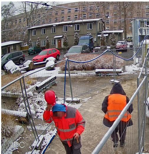
**Figure 6.** Unexpected worker behavior – putting the helmet on behind the detection line
