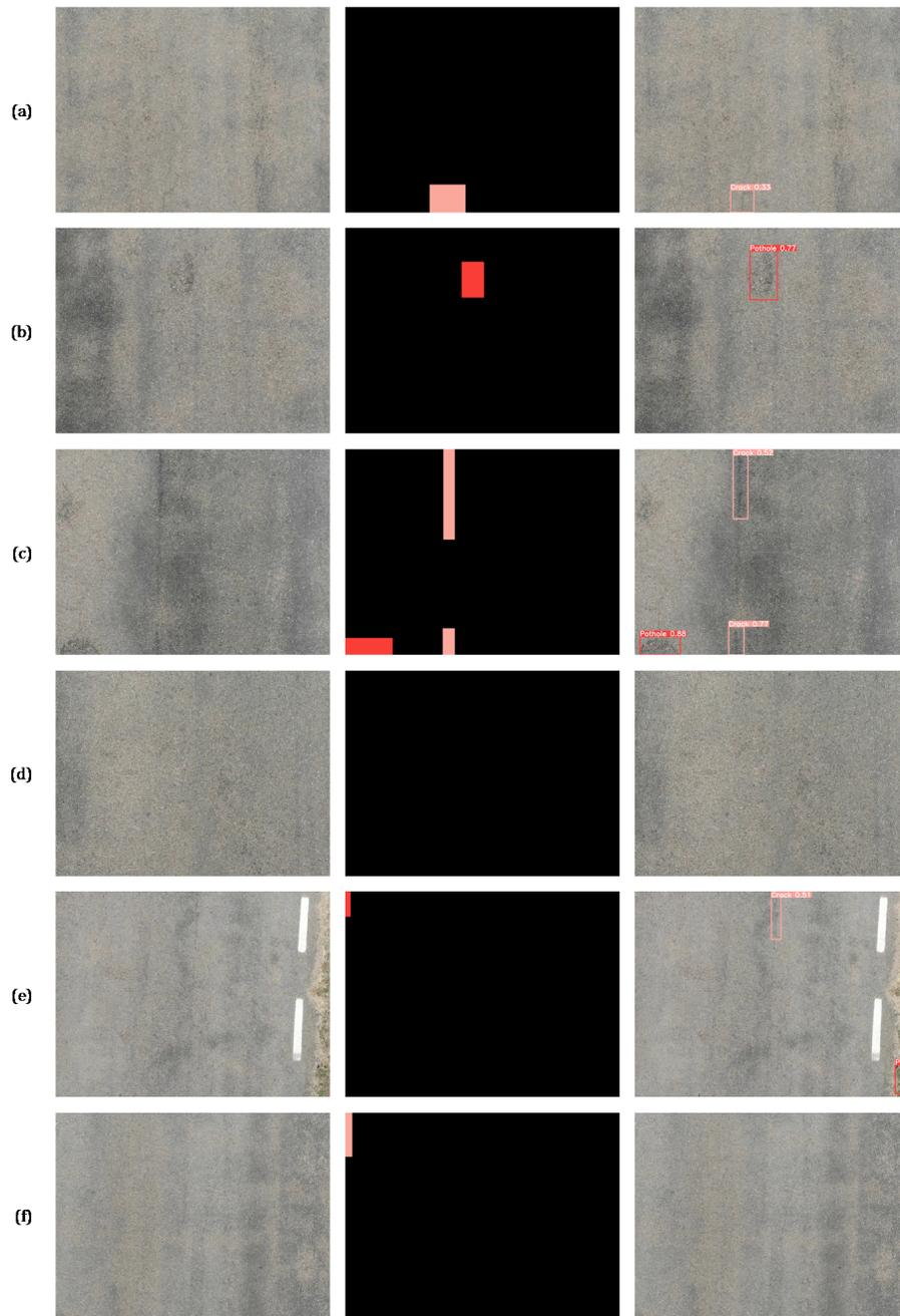
**Figure 4: Automated localization of (i) cracks (pink bounding boxes) and (ii) potholes (red bounding boxes) on UAV images using a small YOLOv5 deep model trained and tested on the dataset [4].**
