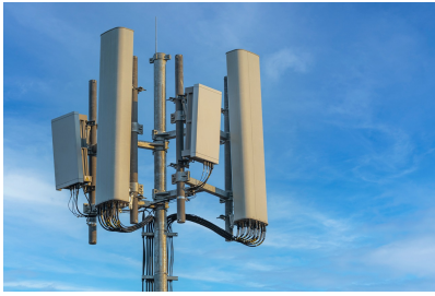
Figure 1: A cellular antenna with sectors that can be tilted.
