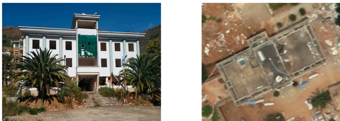
Figure 6. Example of underestimated building damage by visual interpretation of an aerial image. Left: ground photo; Right: aerial image. The collapse of the building is not visible on the aerial image.
